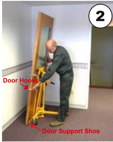
Load the door on the door support shoe and secure with door hooks.
